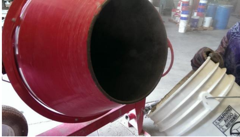
Figure 76 - Charging the mixer
