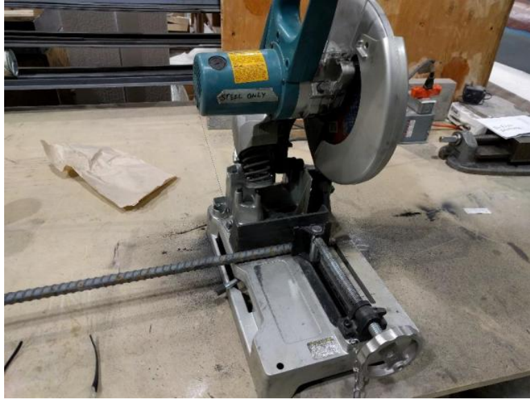
Figure 22 - Cutting reinforcing bar
