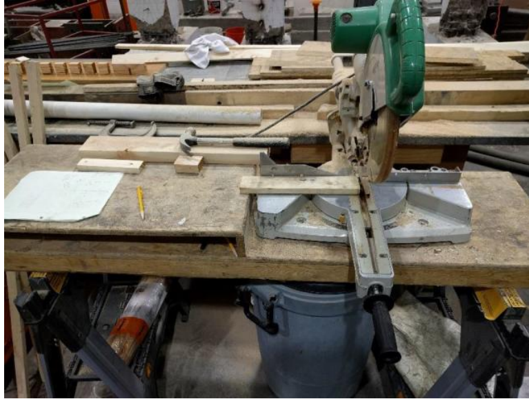
Figure 19 - Cutting wooden blocks for the welding jig.
