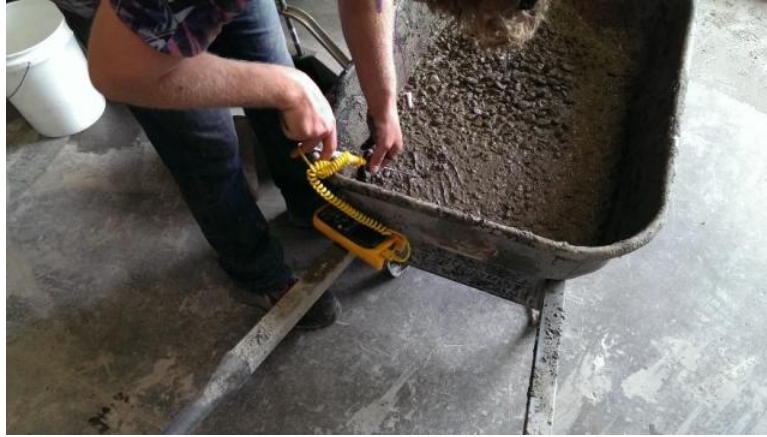
Figure 79 - Placing temperature probe
