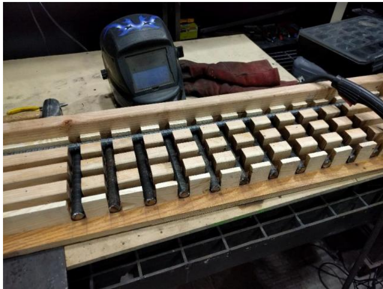
Figure 23 - Rebar layout and welding using the wooden jig.
